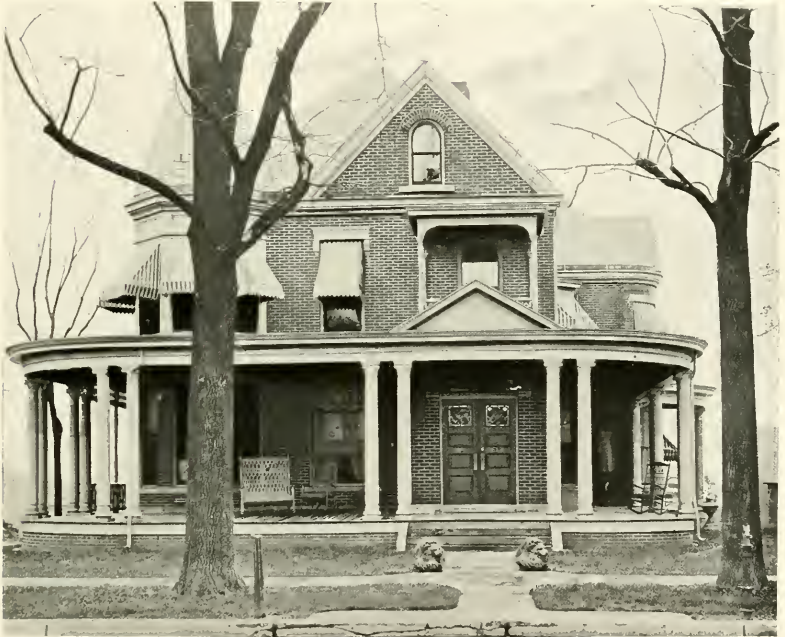
RESIDENCE OF MR. J. A. ROPER.
